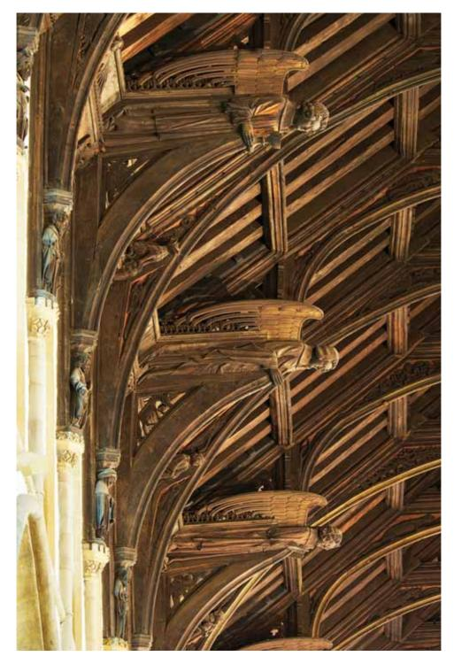
A view along the nave roof at St Mary, showing the alternating angel hammer beams and arch braces.
