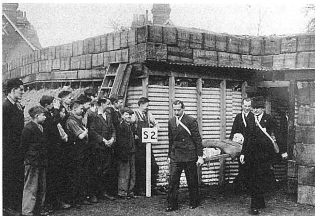
CRATE ESCAPE: Simond's Brewery at Reading used old beer crates to build their air- raid shelter. Note the number of young boys now working at the brewery ( Courage Archive ).
