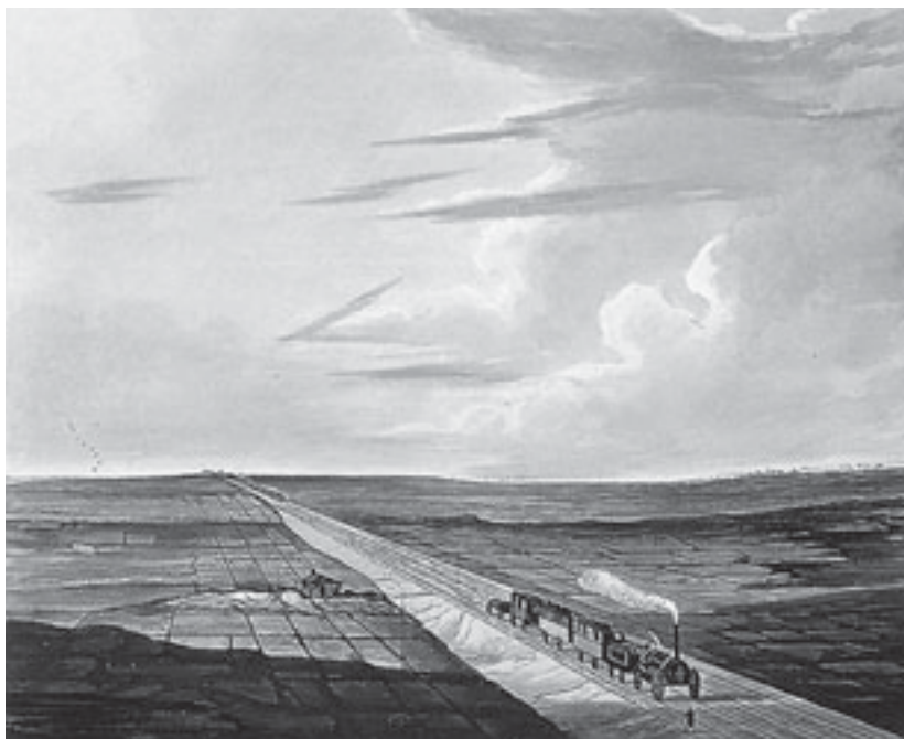
View of the Railway across Chat Moss. Laying a stable trackbed across the deep bog was a remarkable feat of engineering in its time.
