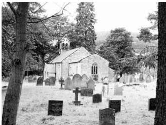
2.13 Hawnby: All Saints Church, restoration 1863.
